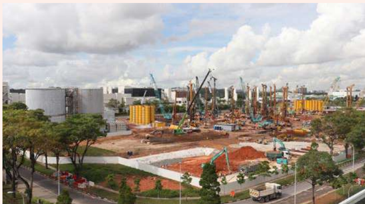
Construction of GlobalFoundries' new Singapore Fab is underway
