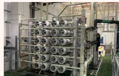
Closed-Circuit Reverse Osmosis system installed in the GF Singapore Expansion facility
